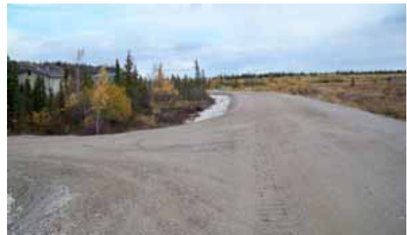
North bypass road completed
